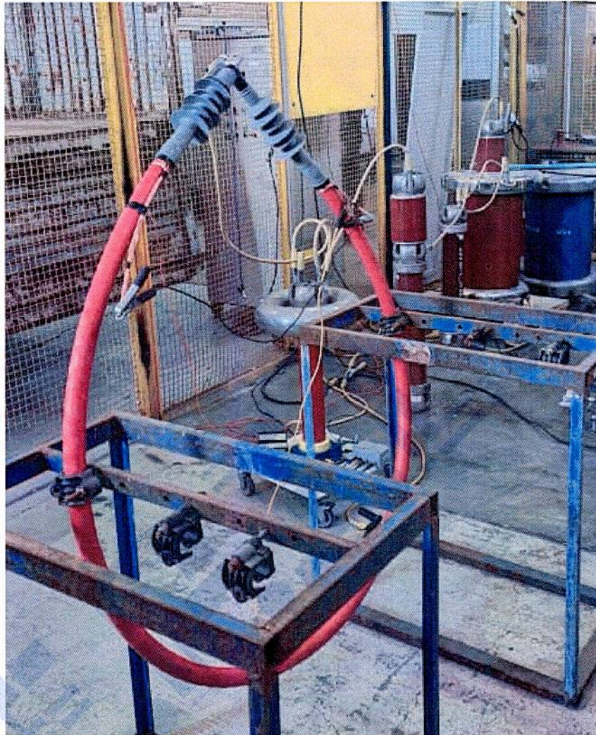
Figure 2. Equipment under partial discharge test
